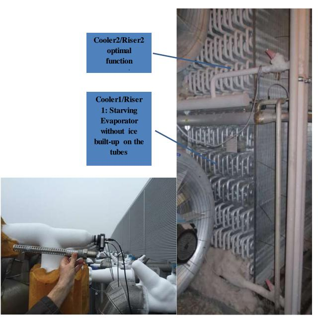
Figures: 18and 19 Sensors applied to four riser pipes at a cold store
